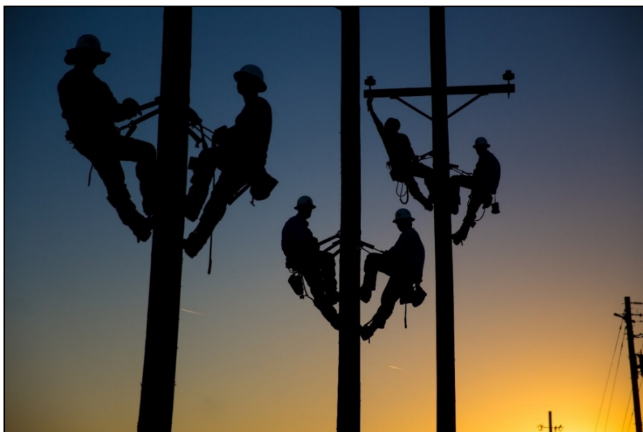
Huntsville Utilities Electric line workers participating in a climbing class.
