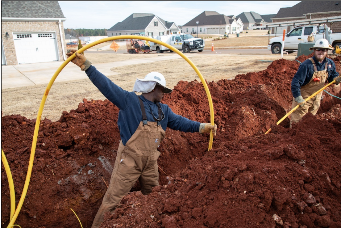
Huntsville Utilities Gas crews installing service lines in a subdivision.
